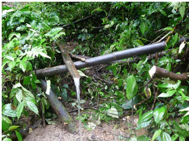
Figure 4: Bamboo "pipe" diverts water from the year-round stream to collection basin.
